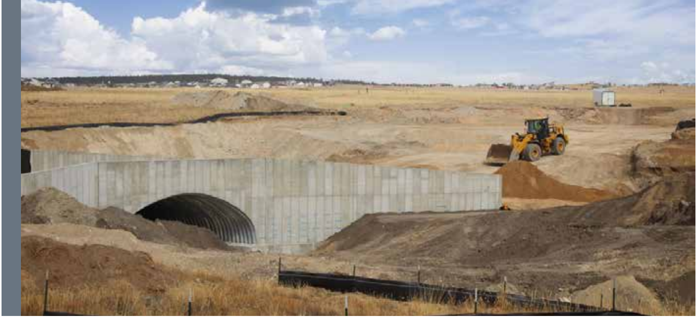
Sterling Ranch Road Crossing of Sand Creek, Oct. 2023.
